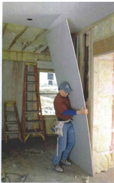
Tilt backward and lift from waist height to position a large vertical sheet.
